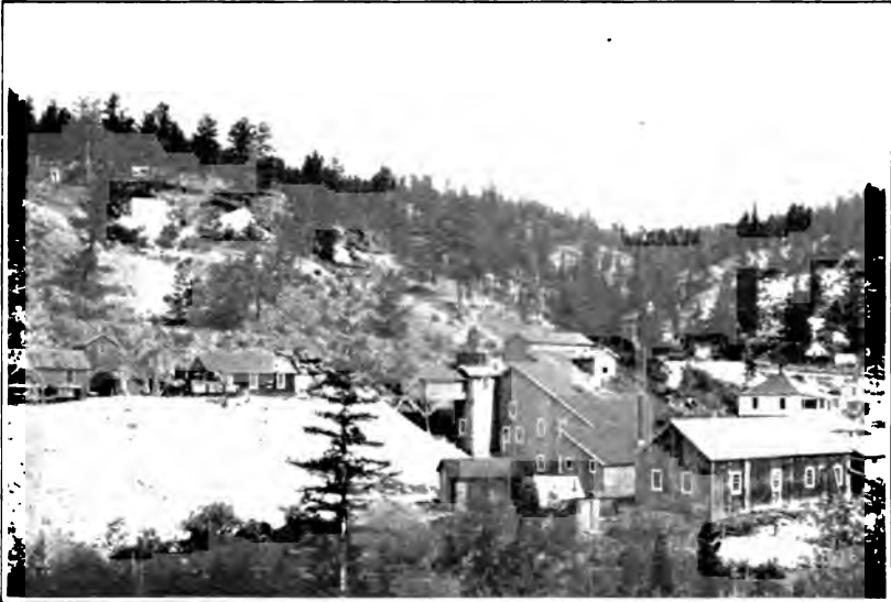
A Concentration Plant, Designed and Erected Complete by Us in Ninety Days
